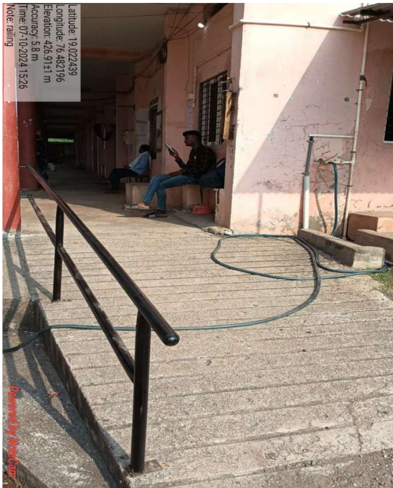
Disabled-Friendly Railings towards Office & classrooms
