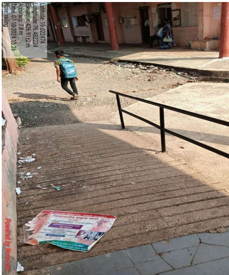
Disabled-Friendly Railings towards Office & classrooms
